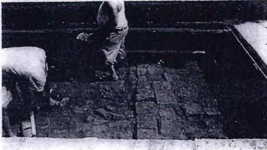
Brick masonry wall all along the foundation wall – view from east
