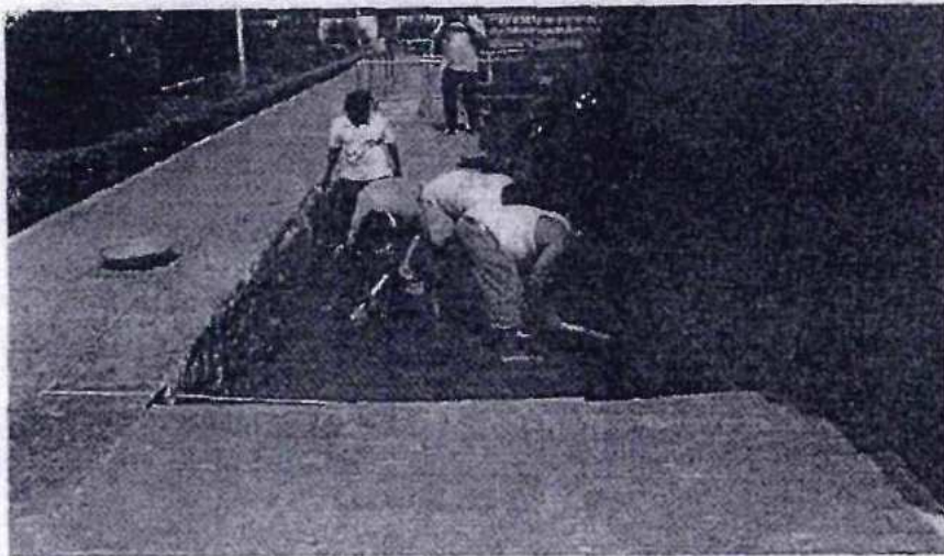
Removal of stone slabs & soil - After - view from south
